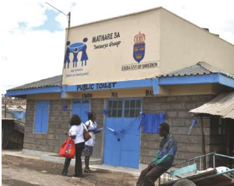
Figure 2: One of the new community sanitation blocks (this one is in Mathare)
