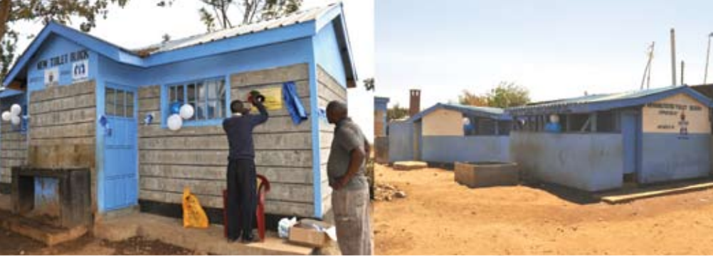
Figure 3: New and rehabilitated sanitation blocks in Njathaini Primary
