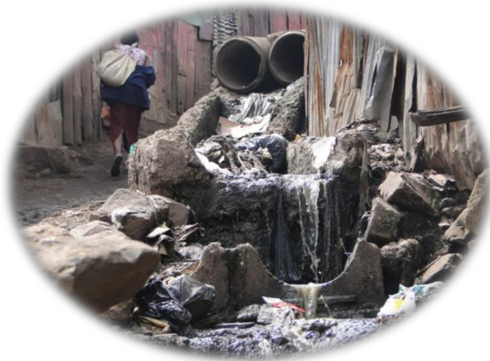
Pic: 4.14: A clogged and incomplete drainage system in one of the slums in the survey area
