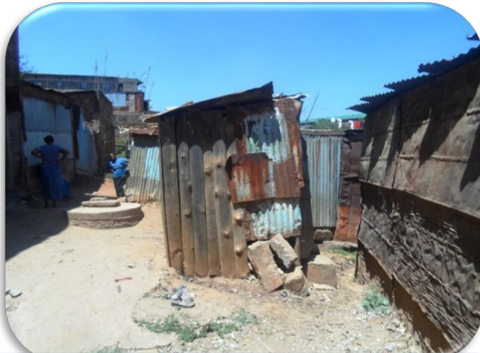
Pic 4.2: A dilapidated pit latrine in Kariobangi North
